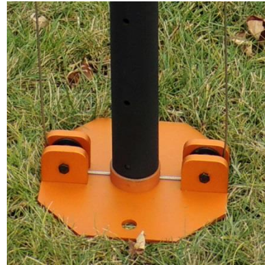
Figure 4-32 After Ensuring Lift Winch is Properly Set Up, Set Next Tube Onto the Raised Plug of the Lifting Plate
