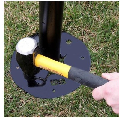
Figure 4-18 Use Hammer to Drive in Stake
