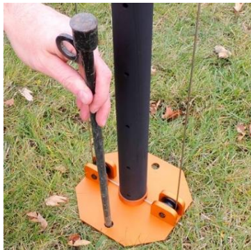
Figure 4-37 Stake the Base Plate
