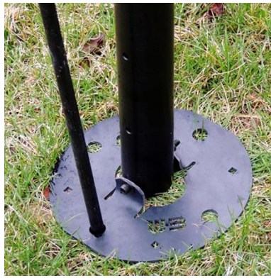
Figure 4-17 Stake the Base Plate
