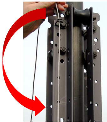
Figure 4-51 Attach the End of the Cable to the Carriage Safety Restraint
