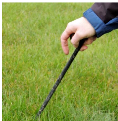
Figure 4-63 Drive Guy Stakes Into the Ground at a 45° Angle Away from the Tripod
